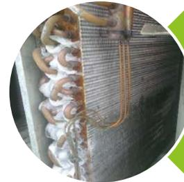
Insufficient airflow can cause a DX coil to freeze and rupture.
