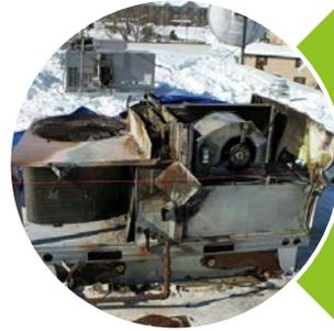
Insufficient airflow can cause overheating of a heat exchanger in a gas-fired unit, and now you have burned your building down.
