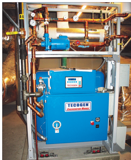
This is the Tecogen CM-75, a CHP system capable of producing 75 kW of electricity while capturing up to half a millions BTU's of free waste heat.
