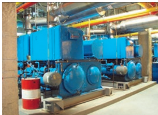
Tecogen Tecochill plant featuring three 400 ton DTx chillers provide cooling and hot water for the capital building of California in Sacramento.
