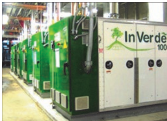
Located on Pier 7 in the heart of Brooklyn, this 600 kW CHP plant provides all the electricity, heating and cooling for the warehouse and offices owned and operated by Phoenix Beverages. This microgrid operates completely independent of the utility grid
