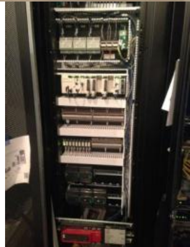
Site microgrid controller + DSO hardware
